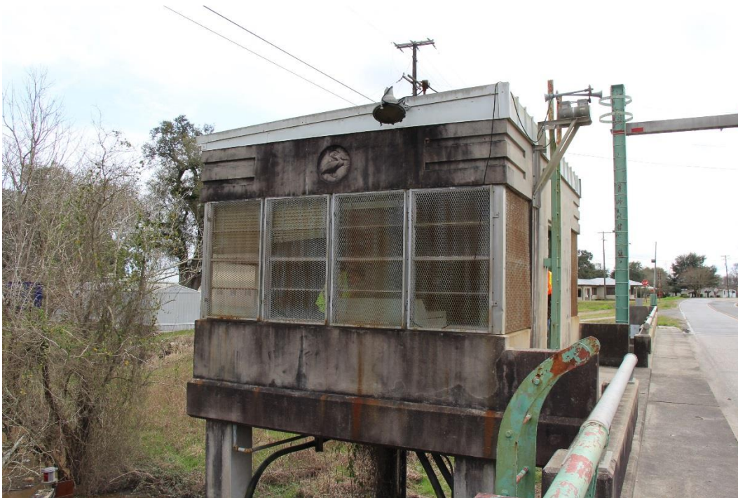
Historic Fabric Photo 4: Operator's House located southeast of the swing span.
