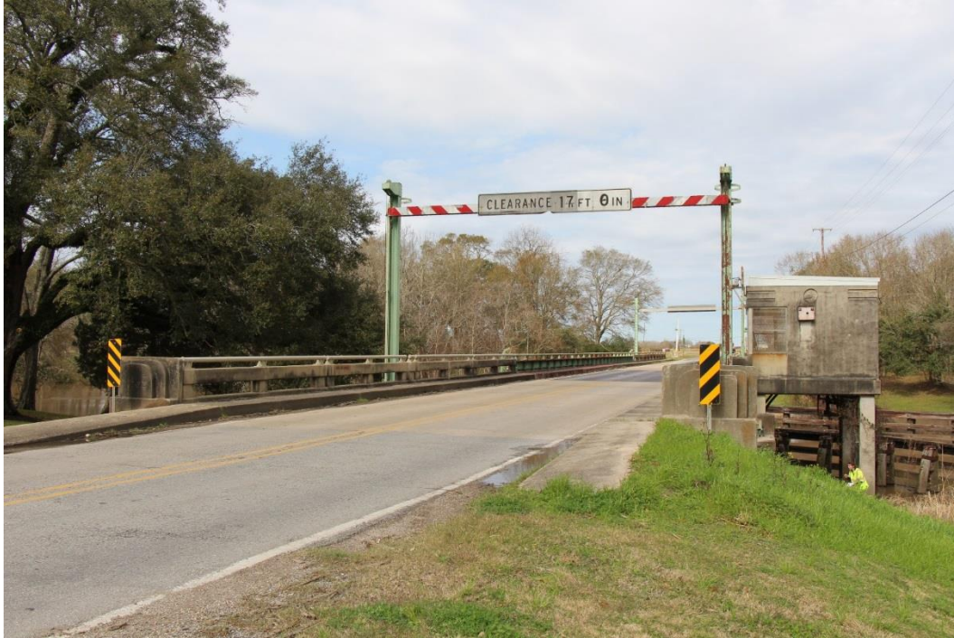
Condition Photo 1: South approach roadway looking north at the bridge. Note traffic barrier gate and towers, and operator's house.
