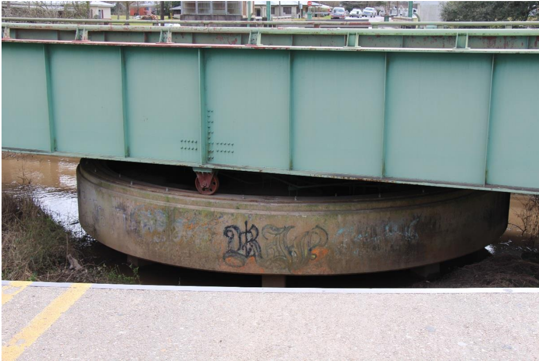
Condition Photo 23: Center pivot bearing and roller assembly; note the graffiti.
